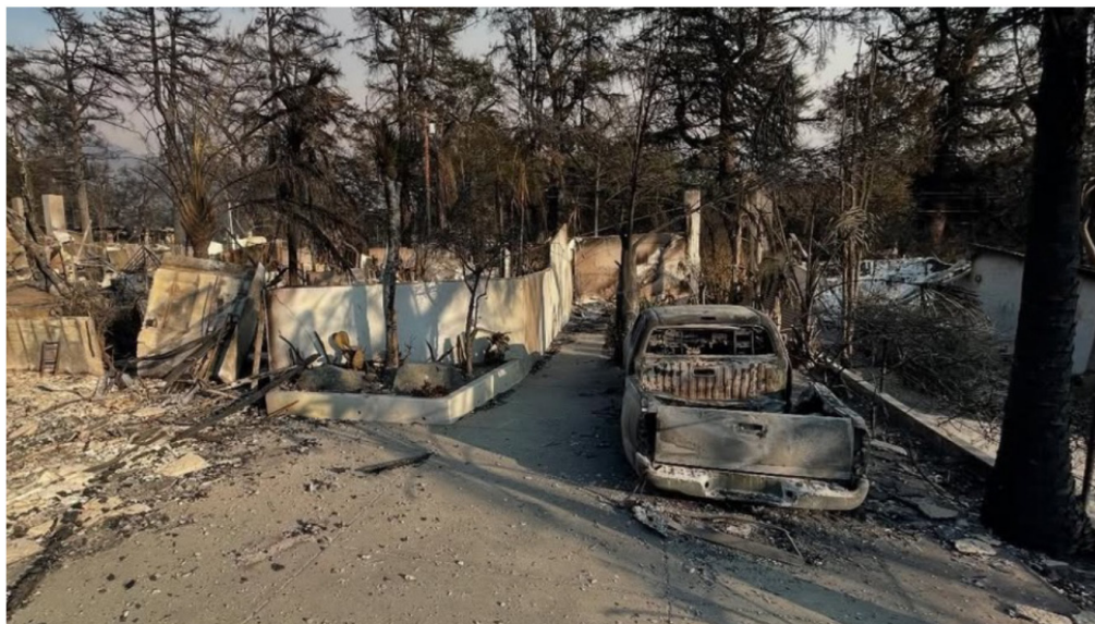
Destruction at Park Planned Homes in Altadena
